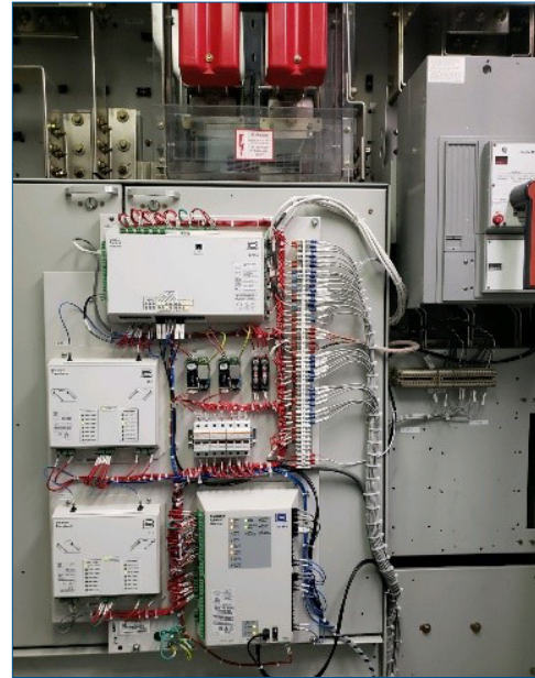
Figure 1 – Updated EX2000 with Panels for the DECS-2100
